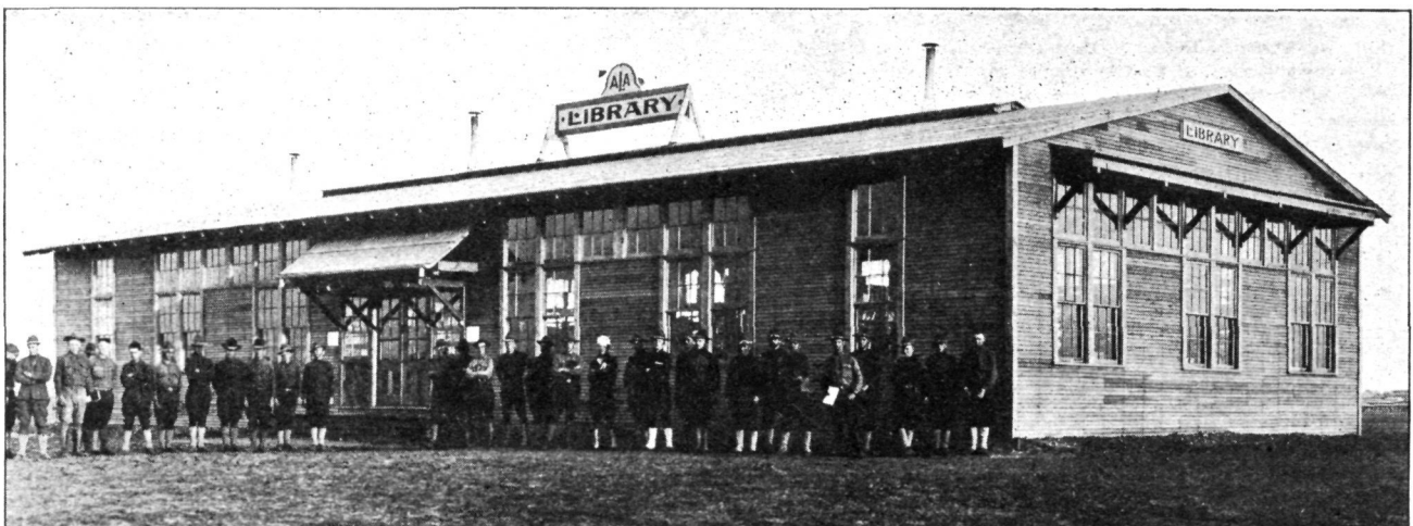
EXTERIOR OF THE LIBRARY AT CAMP DONIPHAN, FORT SILL, OKLAHOMA. NOTE THE WINDOW ARRANGEMENT AND ROOF VENTILATION SYSTEM.
